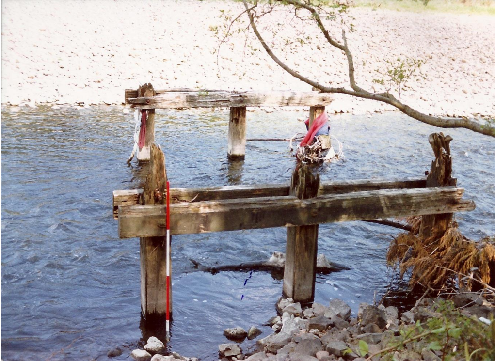
Photograph 1991 of River Tawe railway trestle bridge.
